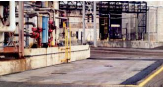
Secondary containment — Truck unloading pad with 3/8" non-skid topping
